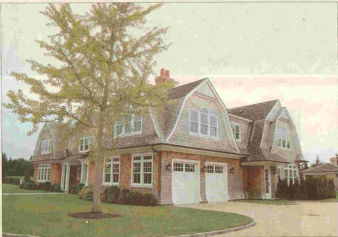
Even from the back view, this Halsey Lane house in Southampton looks just like any other, except it's a whole lot more energy-efficient on the inside and the outside.
